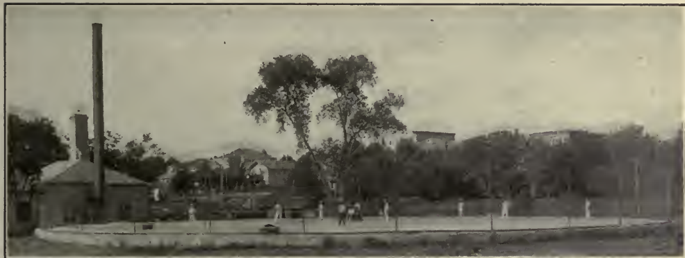
VIEW OF ARKANSAS CITY, KANS., RESERVOIR, SHOWING TENNIS COURTS
